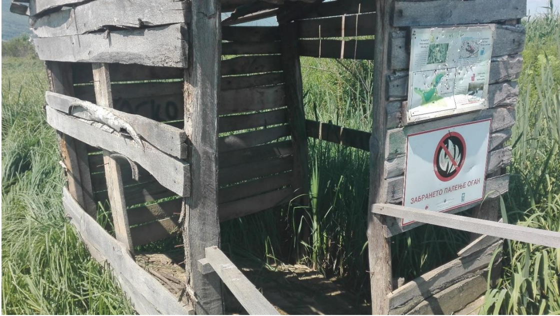
Image no.2 Wooden shack to be reconstructed.
